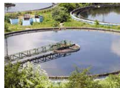
The Oldsmar, Florida, water treatment facility
